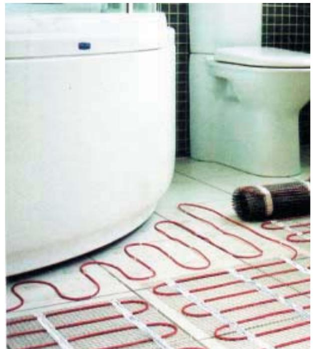
**Cable kit includes:** sheathed cable in mat 500mm wide, floor probe sensor, digital thermostat, lifetime written warranty and instructions.
